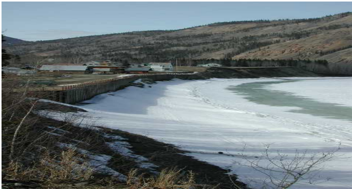
Photo 2: Sheet pile retaining wall along the city of Eagle shoreline protects the bank from erosion. The unprotected high bluff area is in the background, beyond the end of the sheet pile wall; photo courtesy of the Division of Homeland Security and Emergency Management, 2001.
